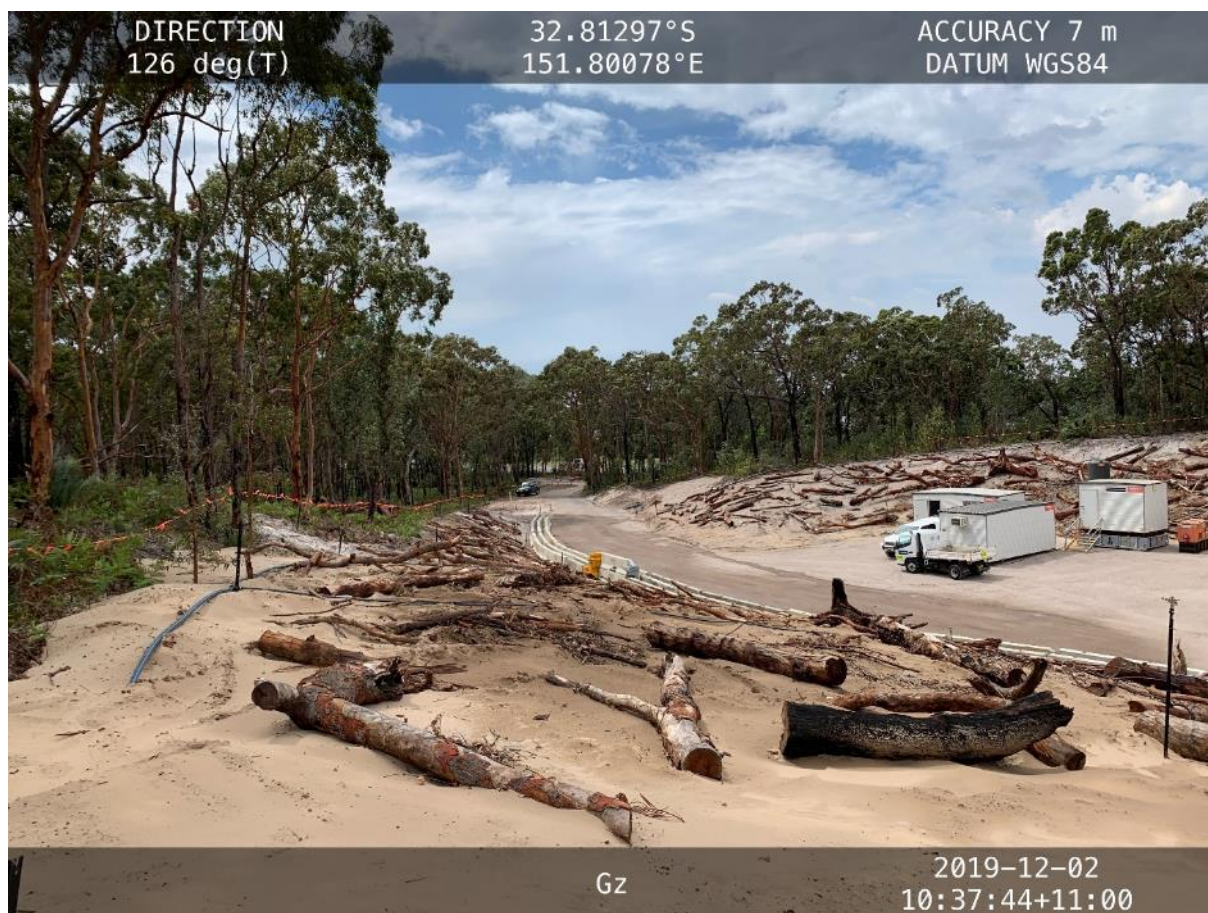
Photograph 2: Jersey Kerb Installation and Cleared Vegetation ground stabilisation looking from site to exit gate
