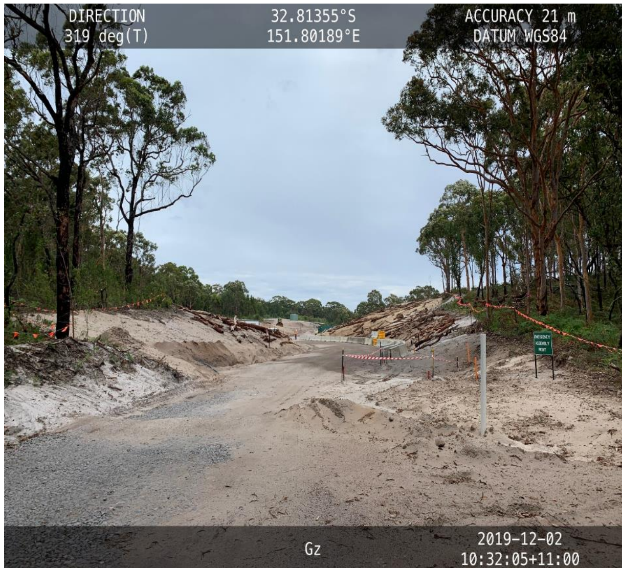
Photograph 1: Jersey Kerb awaiting installation on Cabbage Tree Road and Cleared Vegetation used for ground stabilisation looking into site
