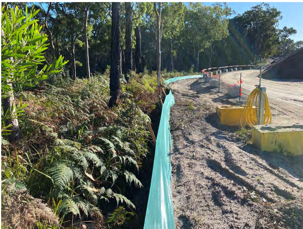
Photo 4 – Installed Frog Fence
