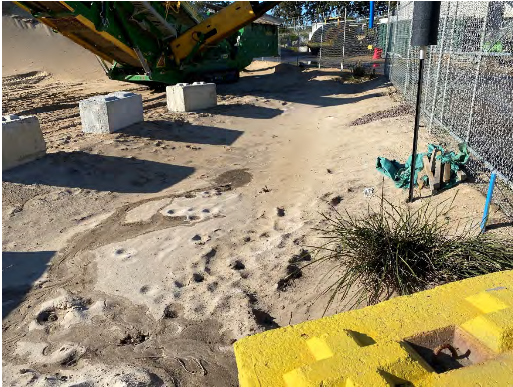
Photo 3 – Sump located behind processing area
