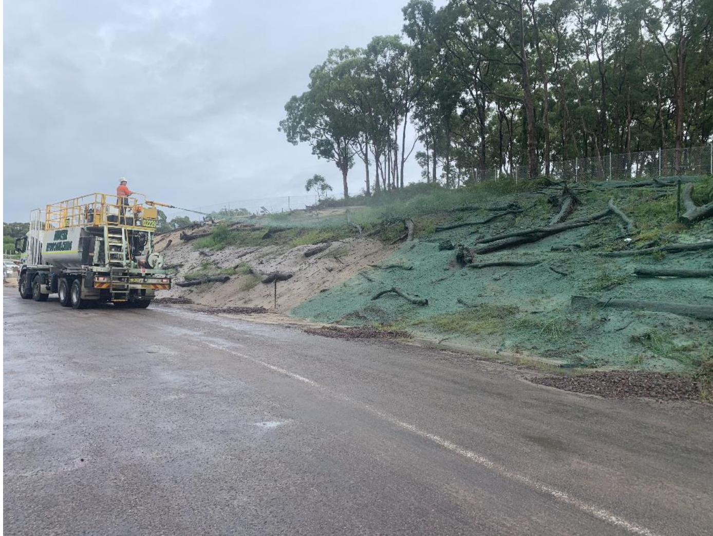
Hydromulch being applied to the batter on the entry road
