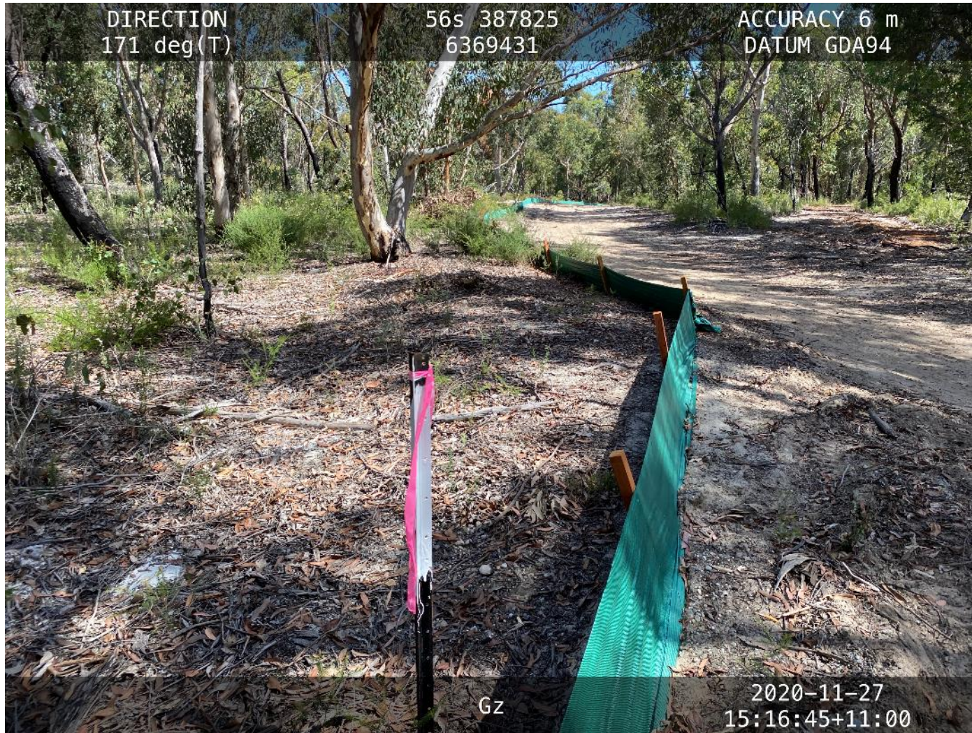
Frog fence installed around Sector 3 and 4
