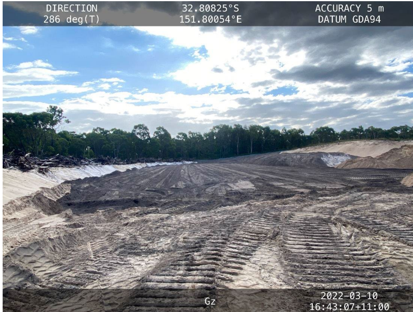
Sector 3A with topsoil spread - next phase will be placement of logs (on left) over the topsoil.
