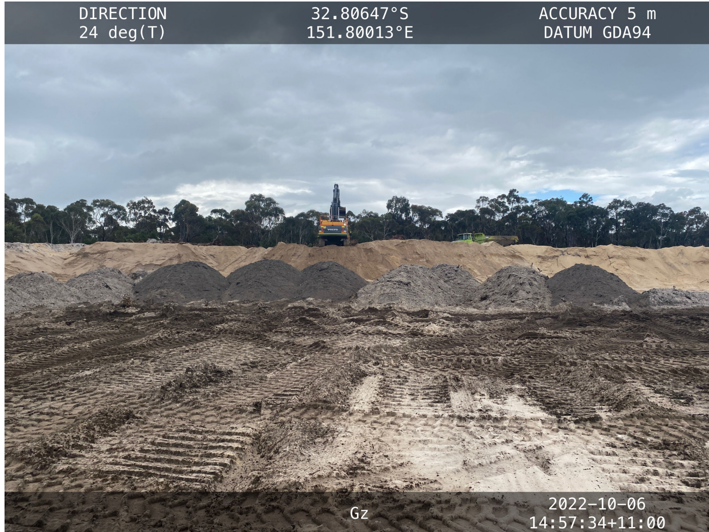
Topsoil stockpiled on the floor of Sector 4B, washplant fines blended into floor.
