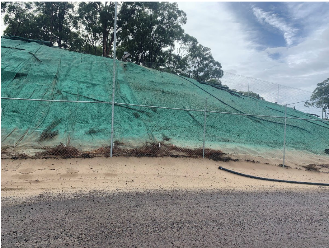
Photograph 2: Temporary batter stabilisation of the batter of Sector 10C adjacent to the Office and access road. Jute matting and hydromulch applied in March 2021.
