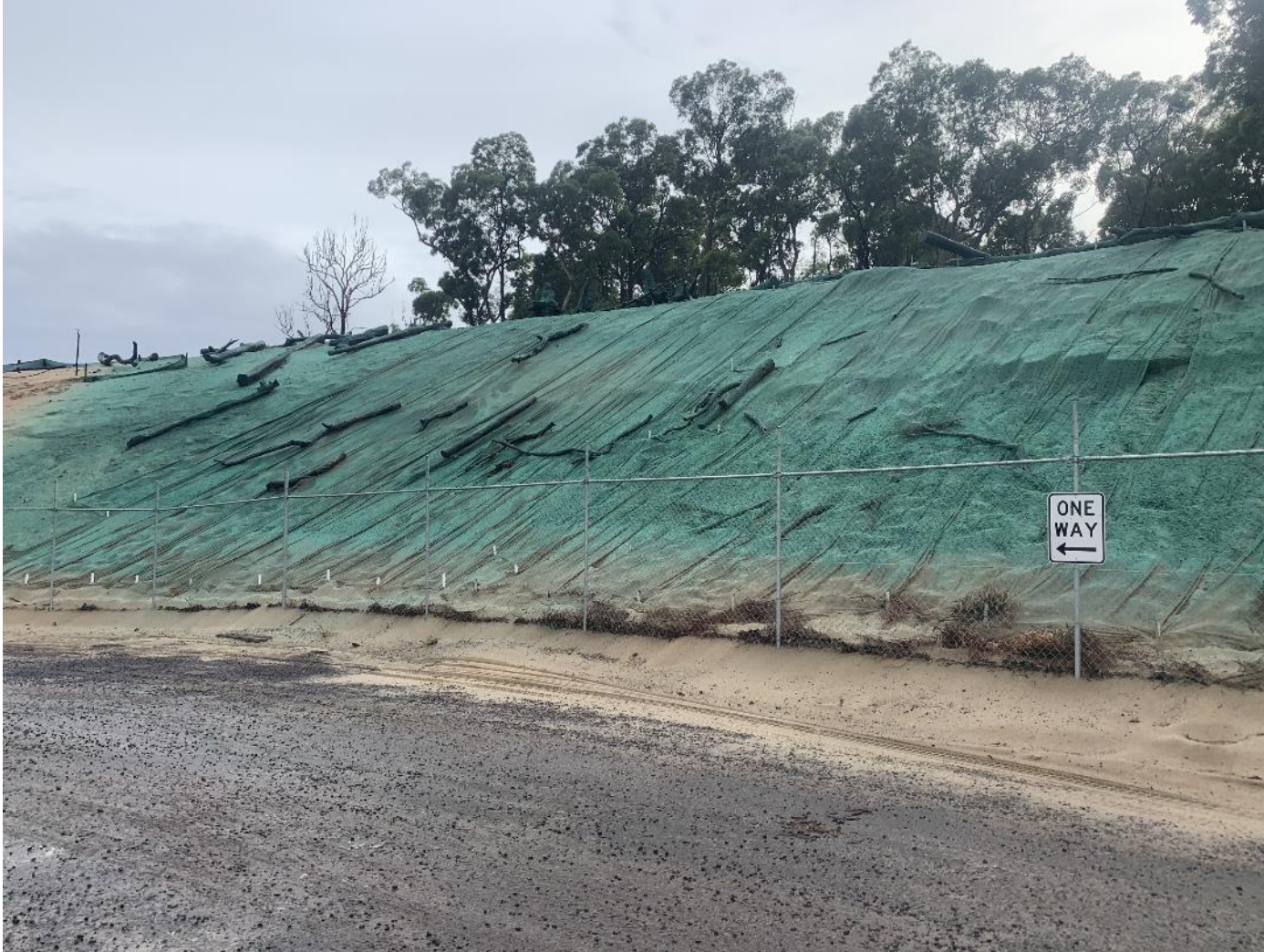
Hydromulch and jute matting applied to the batter adjacent to the office
