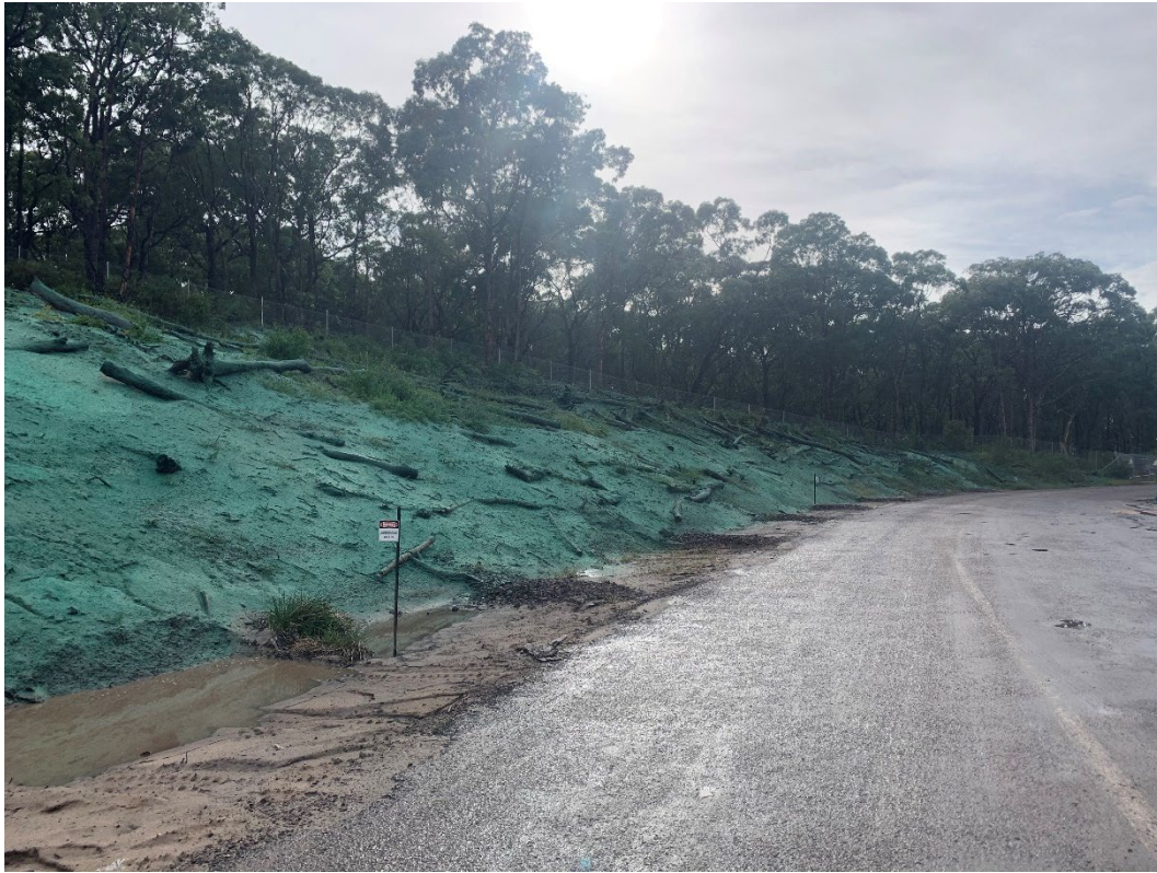
Photograph 1: Temporary batter stabilisation of the batter of Sector 10C and the access road, hydromulch applied, in March 2021.
