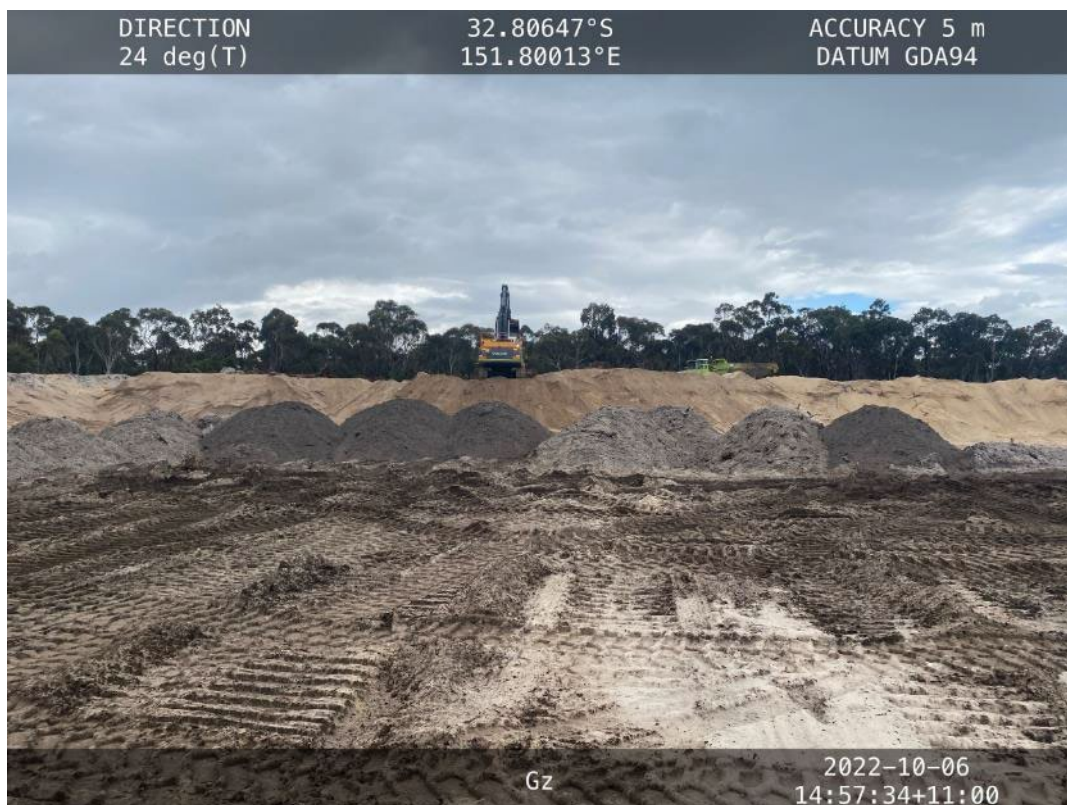
Photograph 6: Topsoil stockpiled on the floor of Sector 4B, wash plant fines blended into floor.
