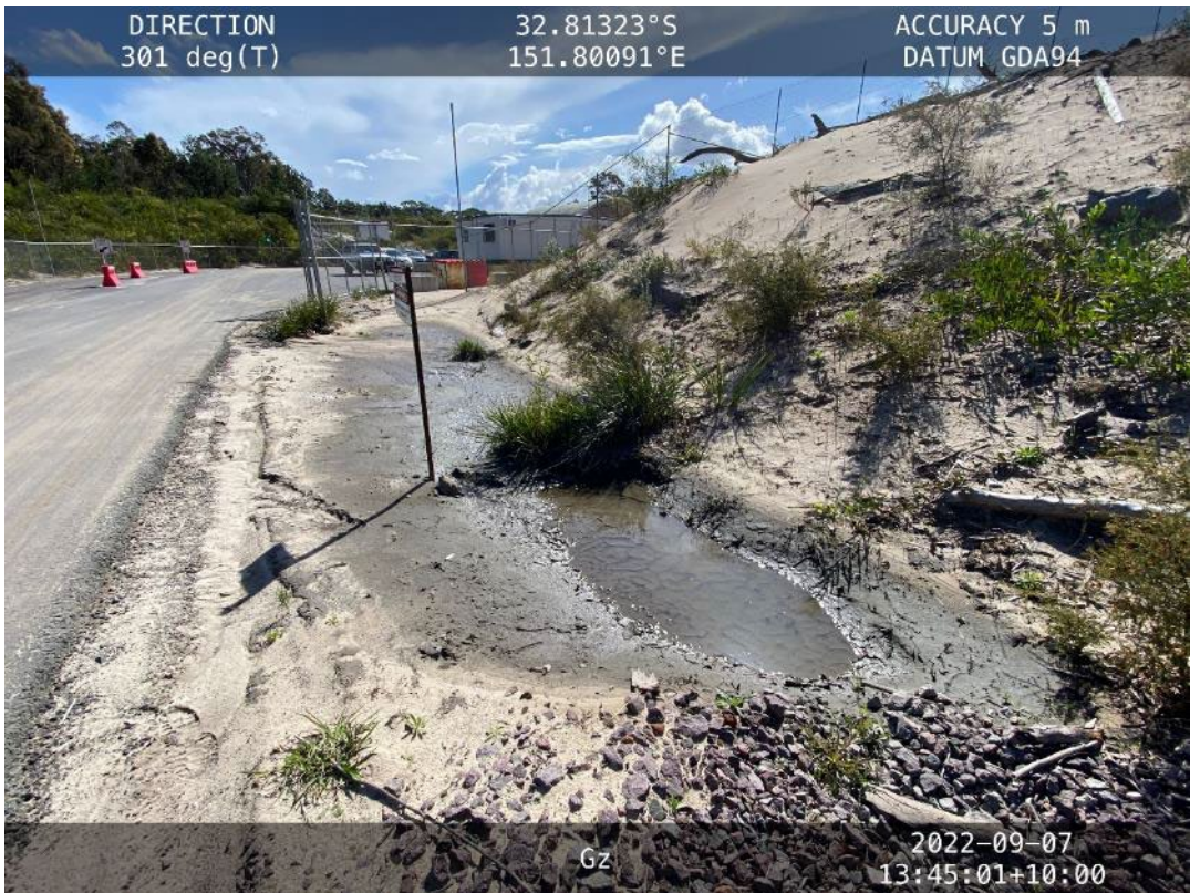
Photograph 3: Roadside drainage with check dams drying following heavy rainfall.
