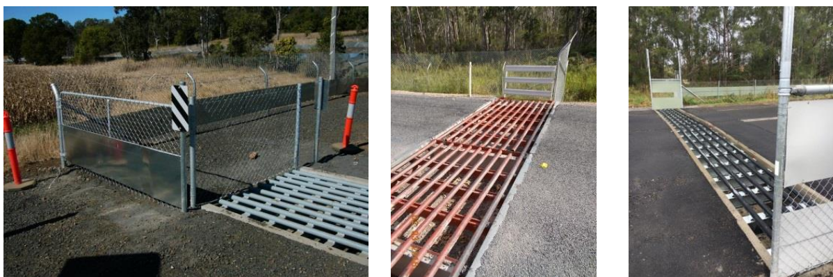
Figure 1. Koala-grid / fence-end configurations. The grid on the far right reflects recent design modifications initiated by NSW RMS as part of retro-fitting modifications on the Gulgan Road interchanges that afford access to the Pacific Highway between Ewingsdale and Chinderah on the NSW north coast.
